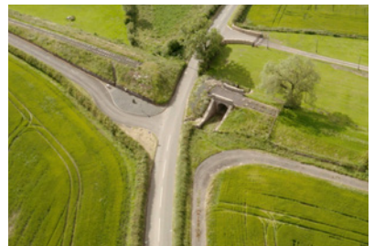
Aerial view of Accommodation Bridge showing the track bed and array of original stone sleepers.
