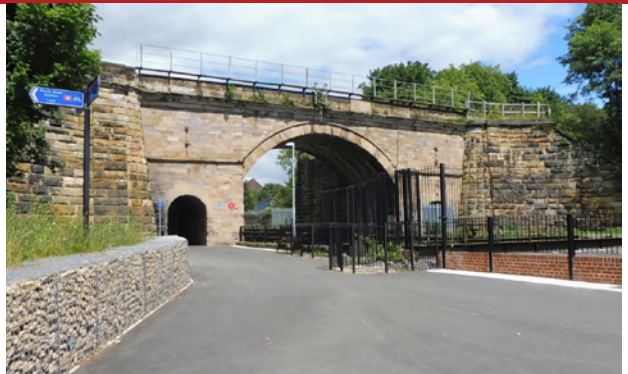
Skerne Bridge, Darlington
