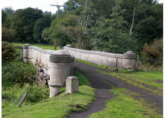
The Skew Bridge on the Haggerleases branch line of the S&DR
